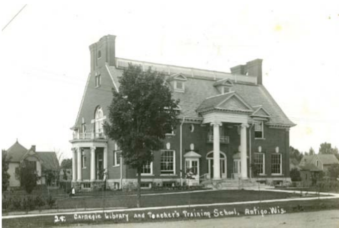
The museum opened as a library in 1905. A teachers' training school initially occupied the second floor. The building is on the National Register of Historic Places.
