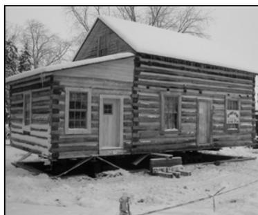
Due to problems with poor drainage, we had to raise the cabin and set it back on blocks so that it was off the ground. This summer we plan to landscape the area around the cabin and the locomotive.
